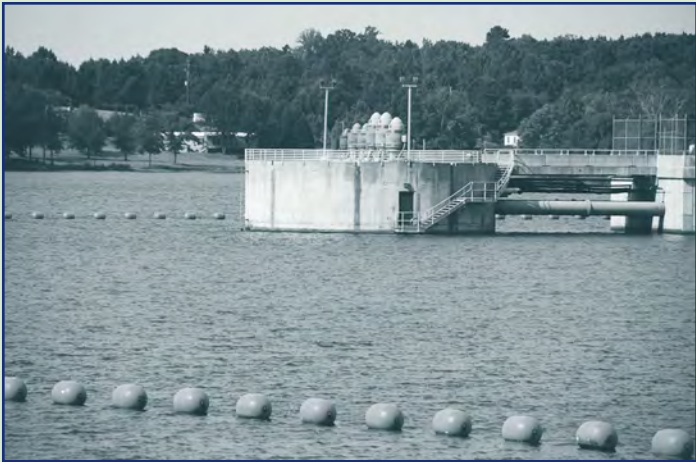
Figure 2b. Many reservoirs are built to hold water that will be used as drinking water. Notice the drinking water treatment plant on this reservoir in northeast Georgia. For more information on water treatment plants, see page 16. Photo courtesy of Babs McDonald.
