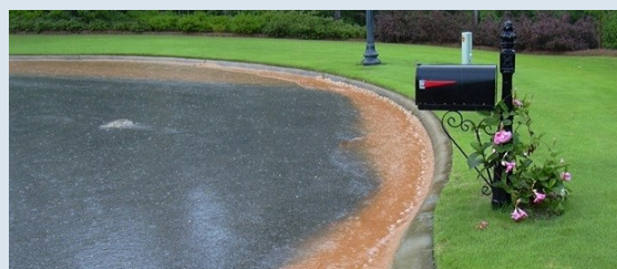
Impervious surfaces like pavement can cause water to flow into streams more rapidly, carrying pollutants such as sediments along with it. Photo by USDA Natural Resources Conservation Service.
