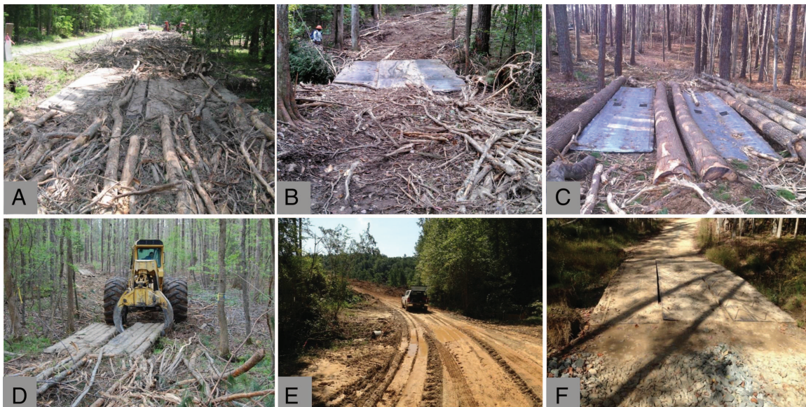
Figure 3. Stream crossing sites. A. DKF1 wood bridgemats on temporary skid trail. B. DKF2 steel bridgemats on temporary skid trail. C. GE steel bridgemats on temporary skid trail. D. HDF1 wood bridgemats on temporary skid trail. E. MC 0.76-m diameter culvert on permanent haul road. F. OC steel bridgemats on permanent haul road. To convert m to ft, multiply m by 3.28.
